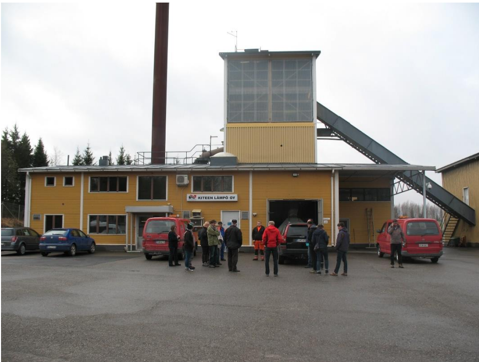
Fig. 3 Next stop was Kiteen lämpö Oy, which is a small thermal power plant in Kitee in the North-Karelia.
